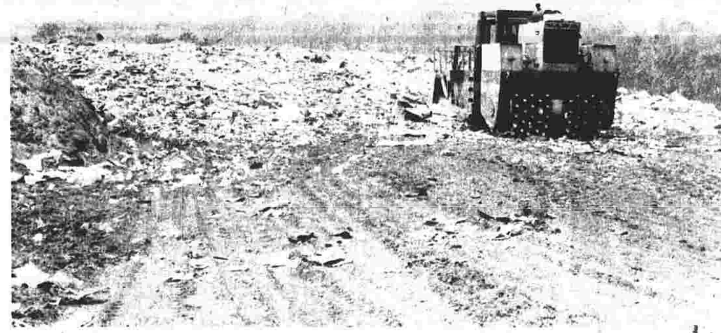
Compacting Manchester landfill
